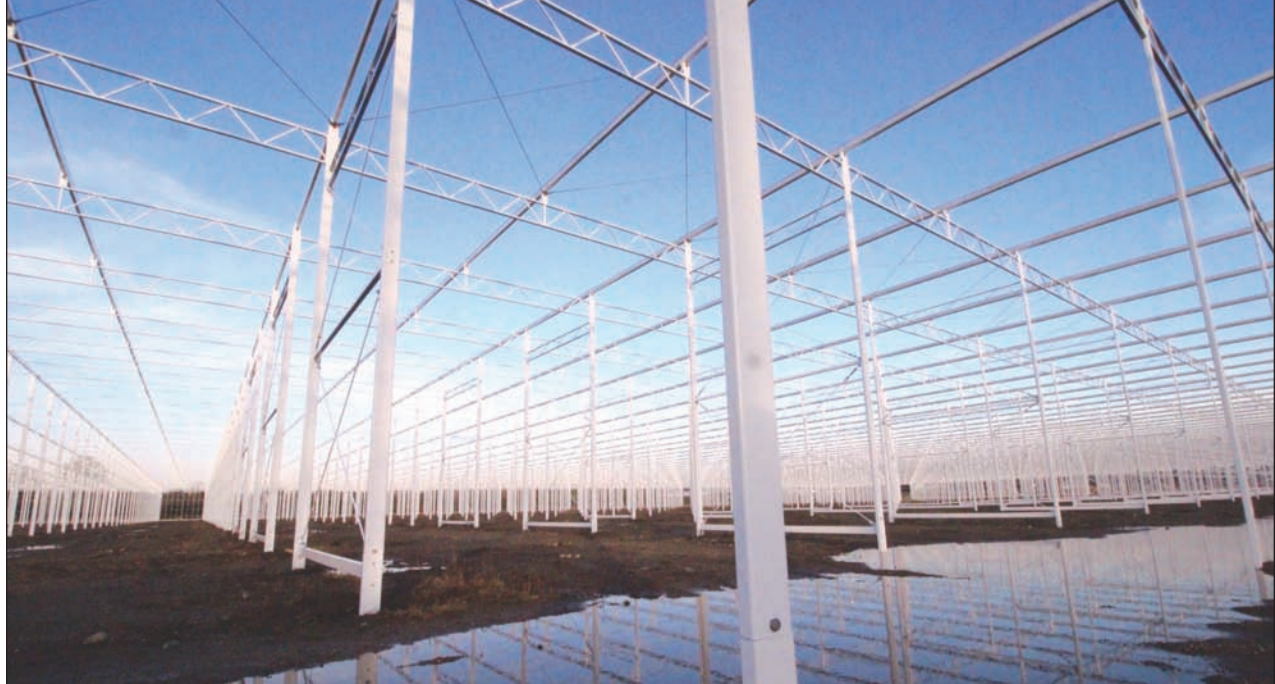
CONTROLLED ENVIRONMENT: Pillars define the framework for the 25-acre greenhouse that when completed will make every day July 27- the best day of the year to grow tomatoes.
